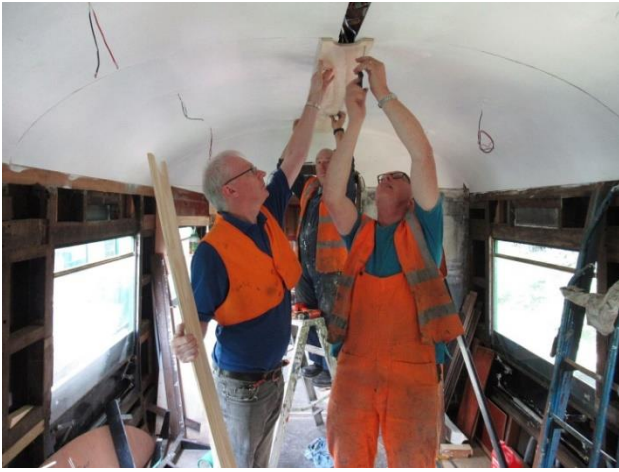
Further down the coach, Mark Humphries does a trial fit of a new side panel,
