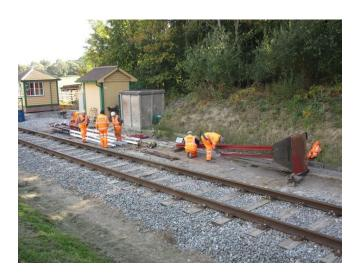
It's 12<sup>th</sup> October, and the S&T gang is at Norden Gates painting some replacement signal posts, which will be erected when there are no train services running.
