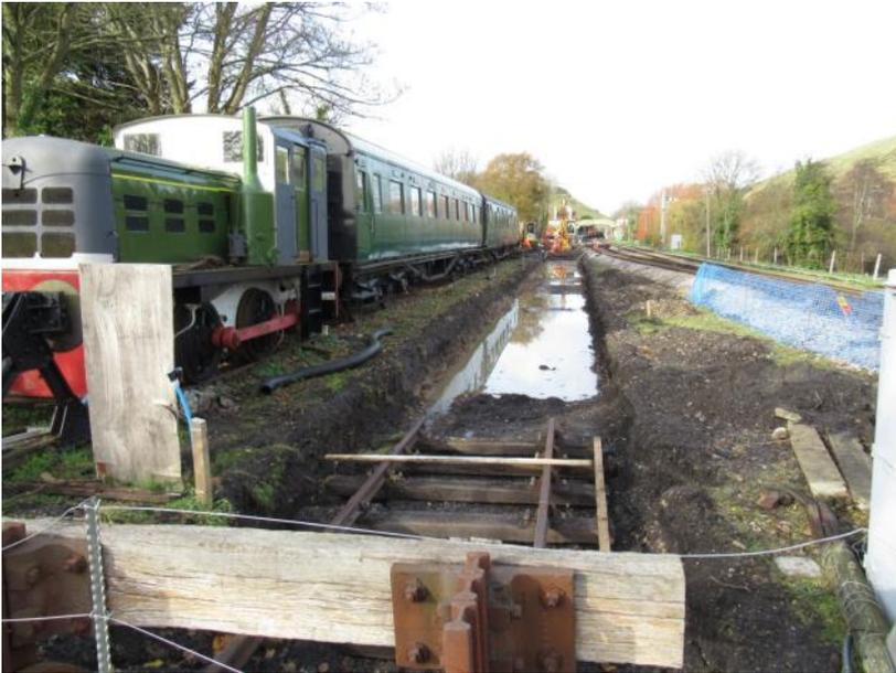
All those works on No 1 siding at Corfe Castle are a precursor for digging an inspection pit for the daily fitness to run exams required for the diesel units for the Wareham service next year.
