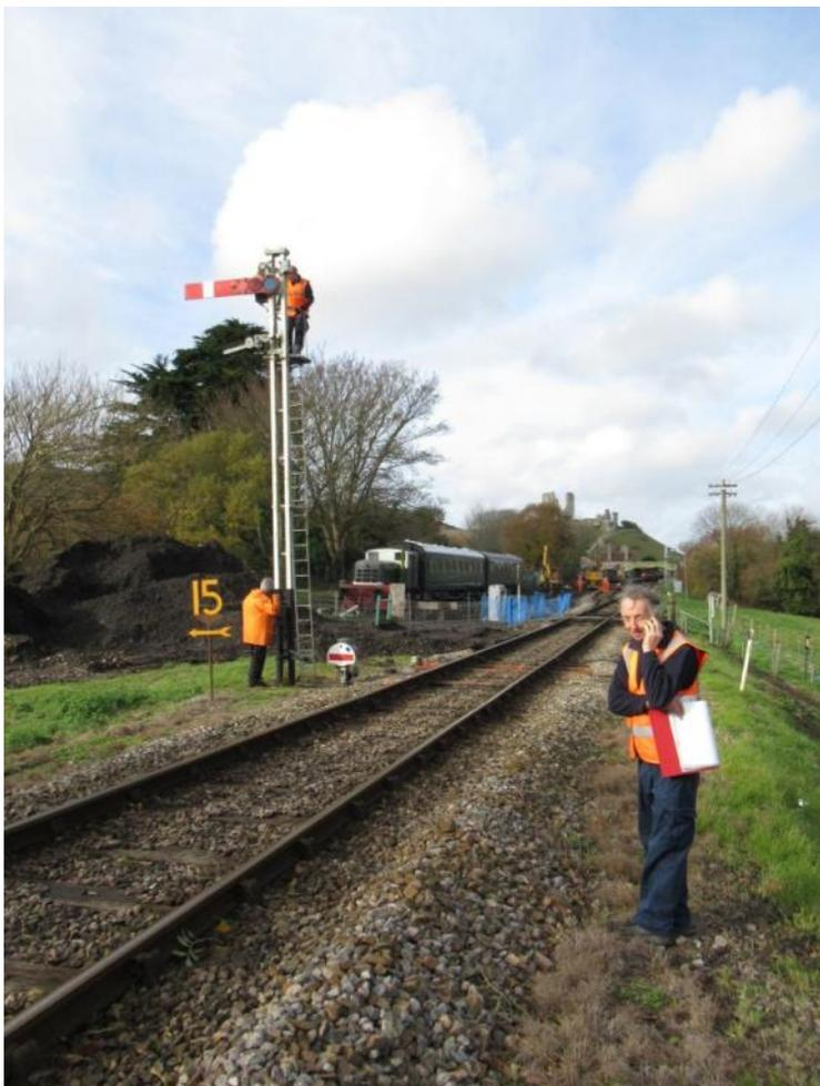
Further on, an attempt is made to check the operation of the Up Home signal. This has to be a limited inspection as it is not possible to operate the signal with the track ahead occupied by the works train.
