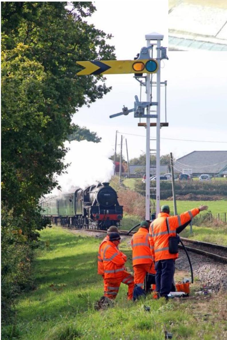
Down the line on 25th October, the Black Five has just left Harmans Cross station towards Swanage and is about to pass the Signal and Telegraph technicians, who have just commissioned the re-located Harmans Cross Up Distant signal.
