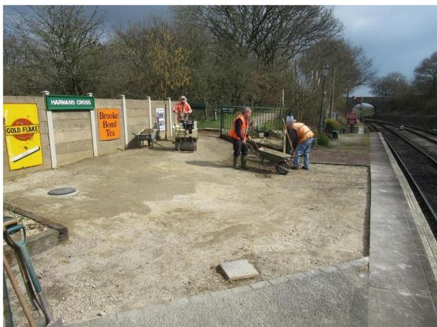
and, on 22<sup>nd</sup> March, the gentlemen from Steve Collins Surfacing are seen first applying a compacted sub-base of Type 1 aggregate to the other patch,
