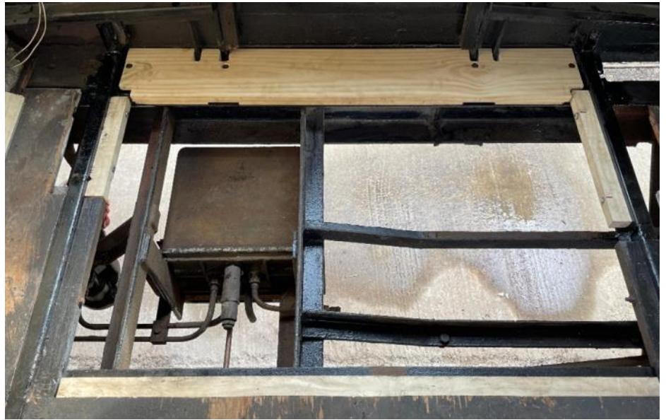
Compartment floor bearers being replaced
