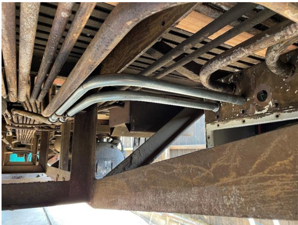
New conduit fitted to replace sections damaged when cable was stolen
