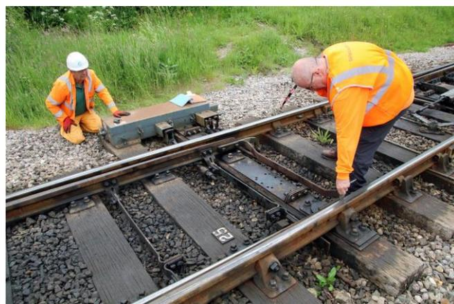
John Tilley checks operation of the electrically-operated points near the crossing, ably assisted by Tony North.
