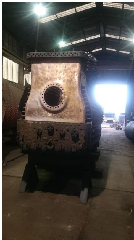
At the firebox rear end, the outer backhead is being cut away prior to fitting a new one. (see next picture also)
