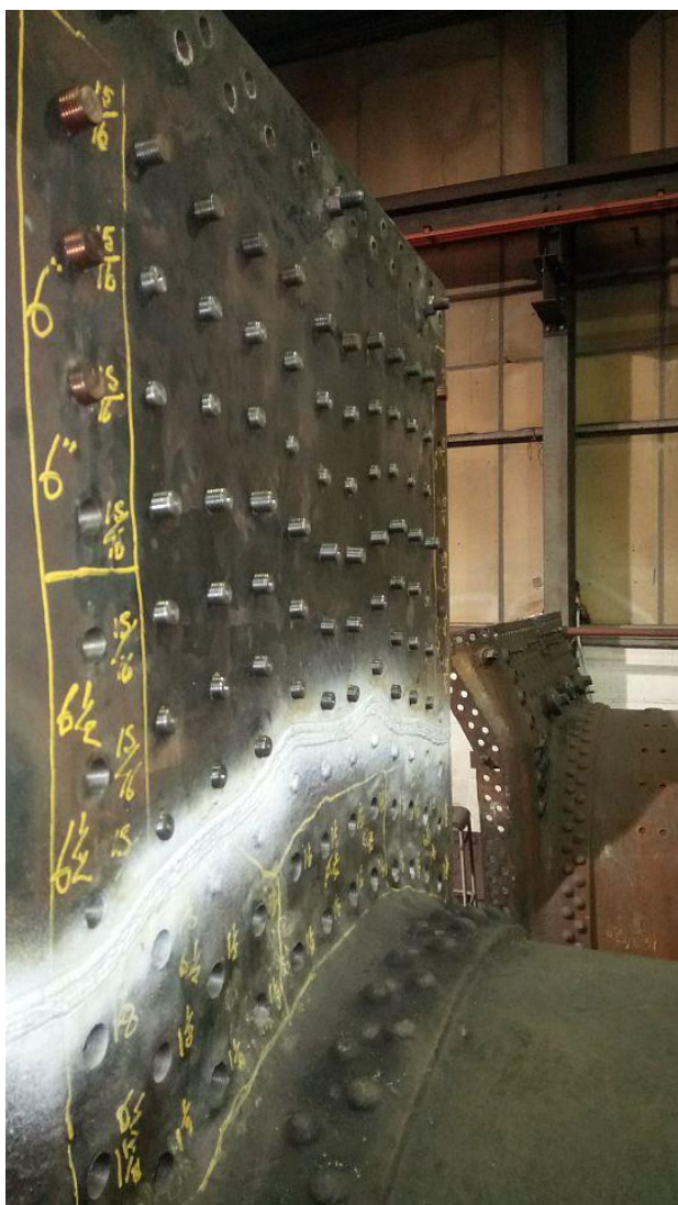
A new lower section of firebox throat plate, that's the bit at the front of the firebox, has been fabricated and welded on, with new stays.
