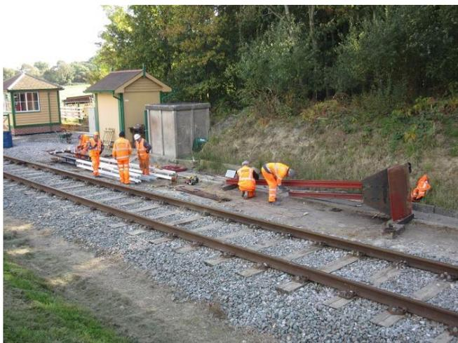
When it is eventually used at Corfe, the bracket will be to the right, carrying a signal for entry to the up platform in the down direction. There's a lot of planning and other work involved before that can happen, though.
