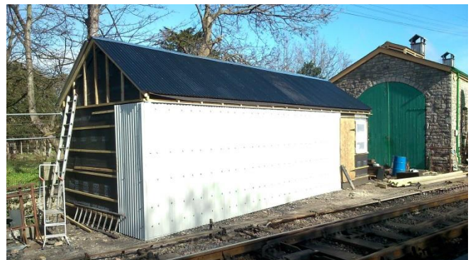
This is the external progress at March 6th.
