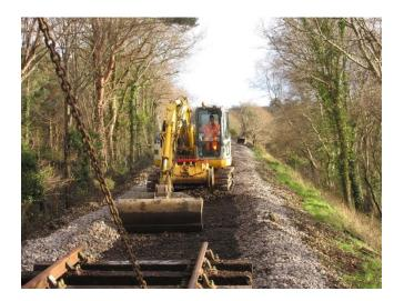
Just some local ballasting and tamping the whole extension left to do to bring the track up to the standard required to run passenger trains. It's nearly there!
